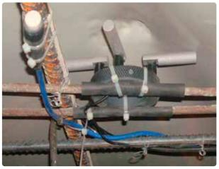
Figure 3. Recommended installation mounted on the reinforcement net. The CorroWatch probe is mounted in combination with an ERE-20 reference-electrode (blue cable).
