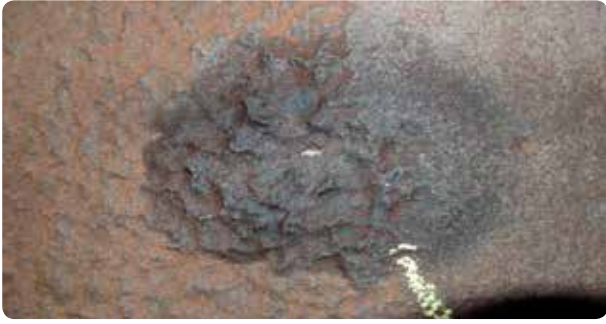
Example of heavy underside corrosion on tank cut out from a tank bottom
