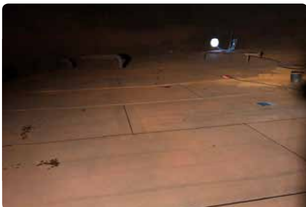
Tank bottom seen from the inside
