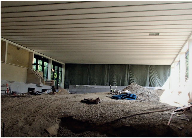
The renovation project well under way.
