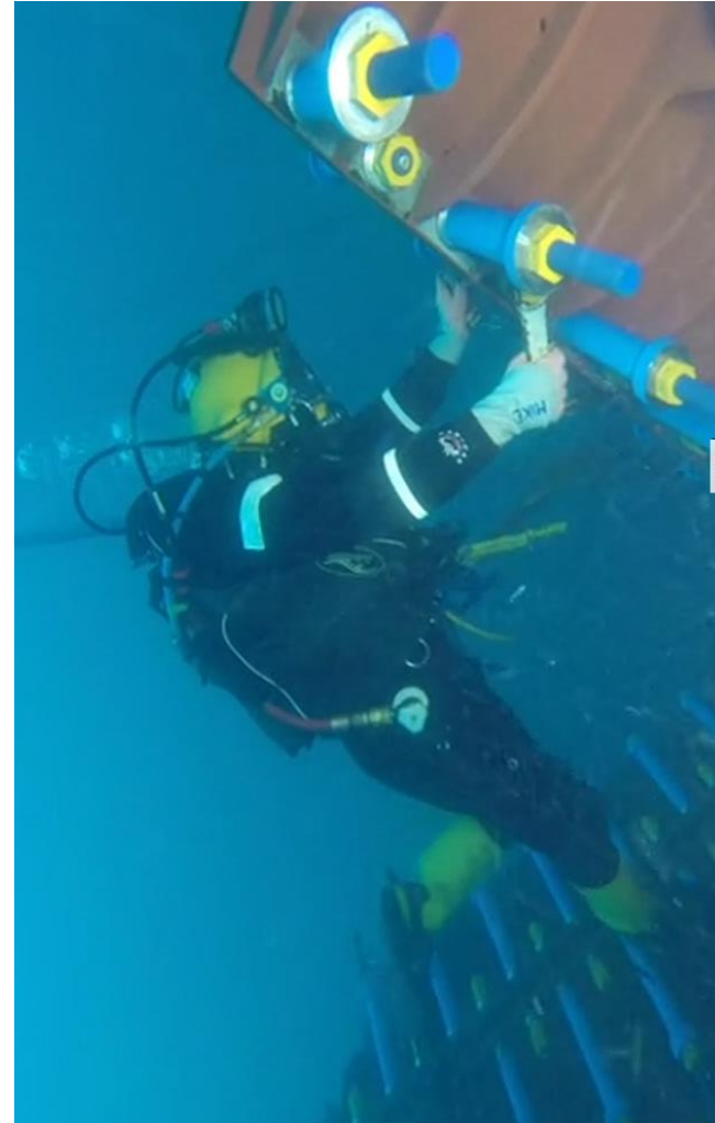
Clamp installation on oil rig. Source: ing.dk
